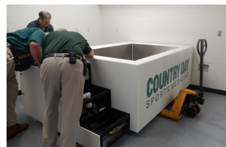
fig. 6 - Leveling the CRYOTherm
